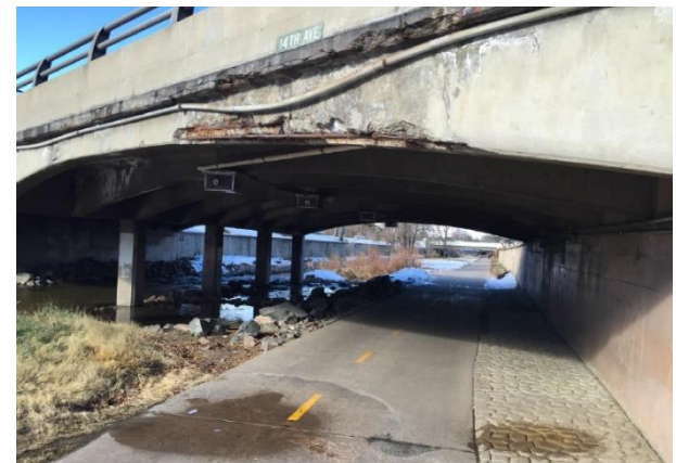
14 th Ave over Cherry Creek – bridge beam concrete failing directly above trail.
