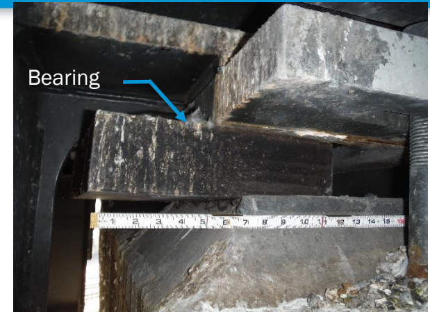
Park Avenue Viaduct – unanticipated horizontal movement in support (bearing). Could lead to bearing failure and 4" vertical drop.
